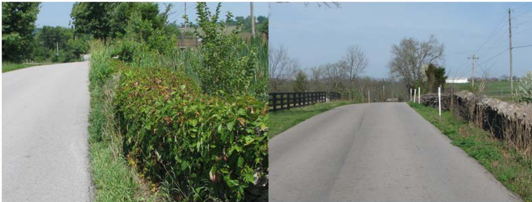
Before and After Photos of the Rock Wall on Clear Creek Rd.
