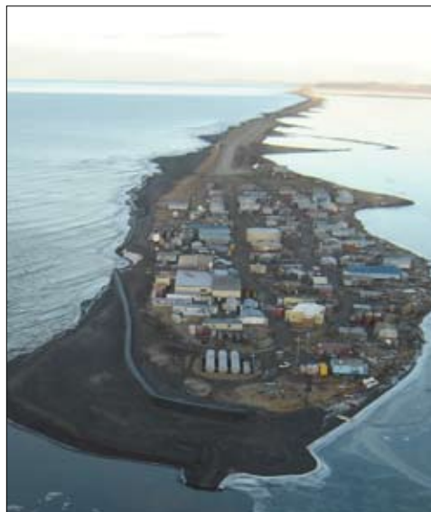
Years of erosion has left almost no buffer against waves invading the village of Kivalina. (Courtesy photo)
