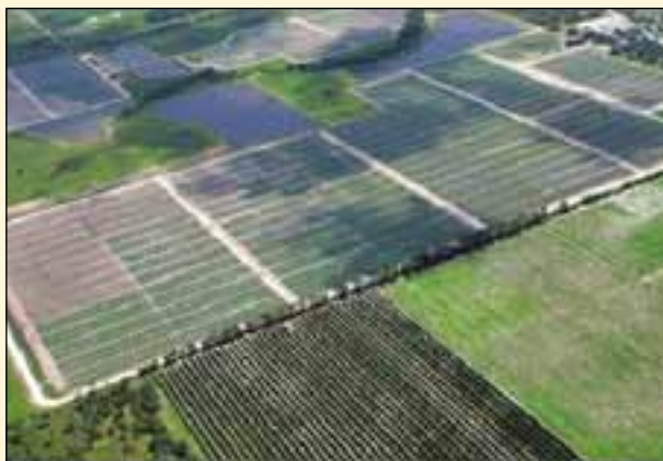
Systems Integration for Solar Technologies. A 25-megawatt photovoltaic system in DeSoto, Florida, generates enough electricity annually to power about 3,000 homes.
