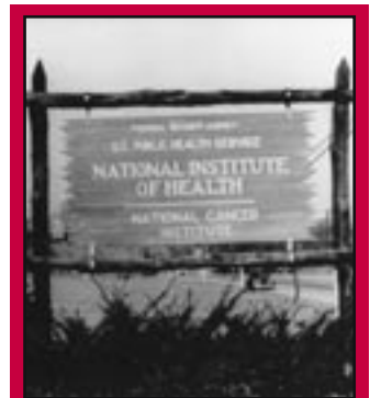
Original road sign that reflects NCI as the only Institute of the NIH
