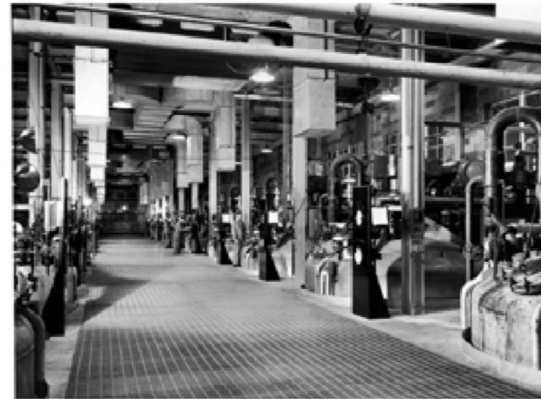
Upper part of fermentors (tanks) used to produce penicillin and vitamin B12.
