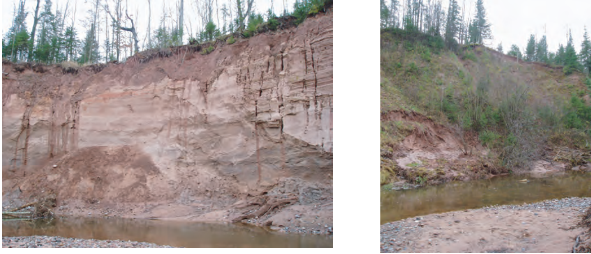
Figure 14. Photographs of site 16.4: the vertical bluff face between cross-sections 4 and 5 and upstream slump between cross-sections 2 and 3 after the October 2005 flood. See figure 4a for cross section locations. Photographs by C. Storrar, November, 2005.
