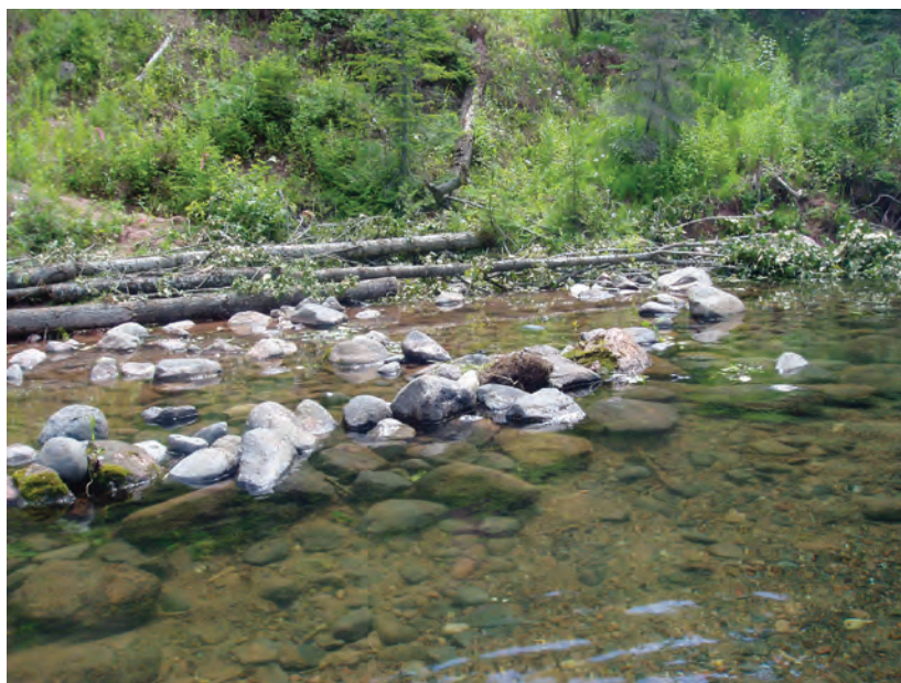
Figure 19. July, 2004 photo of rock dam and cabled logs at base of bluff at site 14.4.
