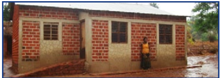
Jesca poses in front of her family's new home during construction.
