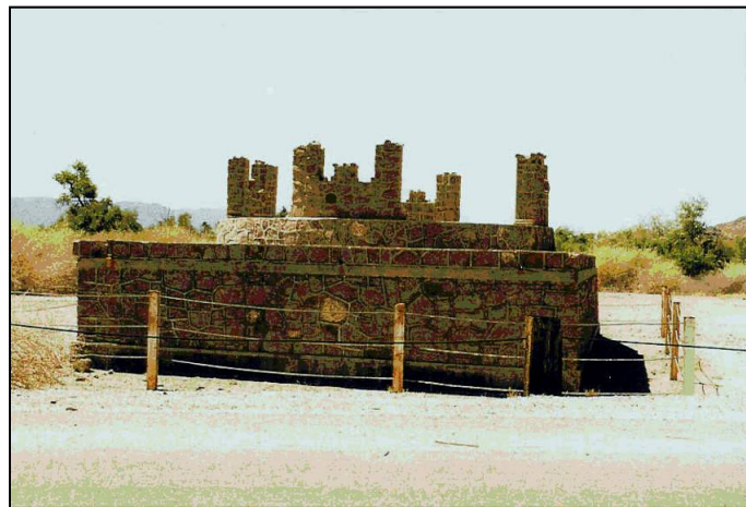
Figure 3-16. Elaborate Paint Locker Constructed by Italian Prisoners of War (Source: Peyton 2000)
