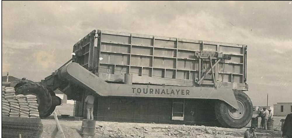
Figure 4-7. Tournalayer Machine Lowering Form Over Interior Building Frame
