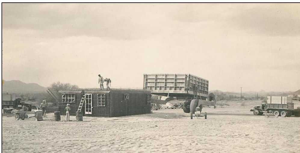
Figure 4-6. Tournalayer Machine Approaching Interior Building Frame with Form
