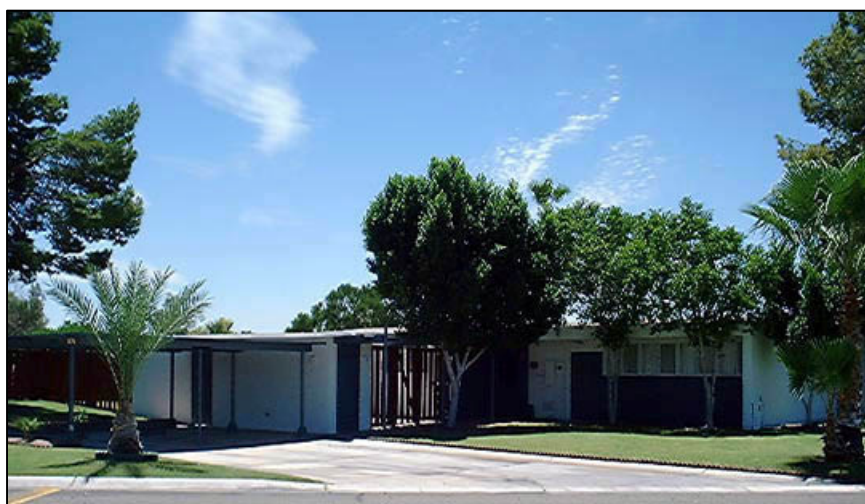
Figure 4-3. Building 976 at YPG, Neutra and Alexander Designed Residence (Colorado Housing Area/3-BR/Type A/O5, W5) (Source: https://www.housing.army.mil )
