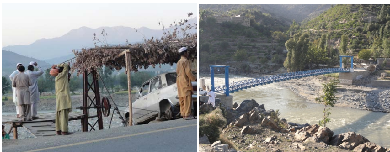
At left, residents use an automobile to power a cable to carry one person at a time across a river in KPK. At right, a program-funded bridge allows for quick and safe river crossing. (Photos by OIG, October 2011)
