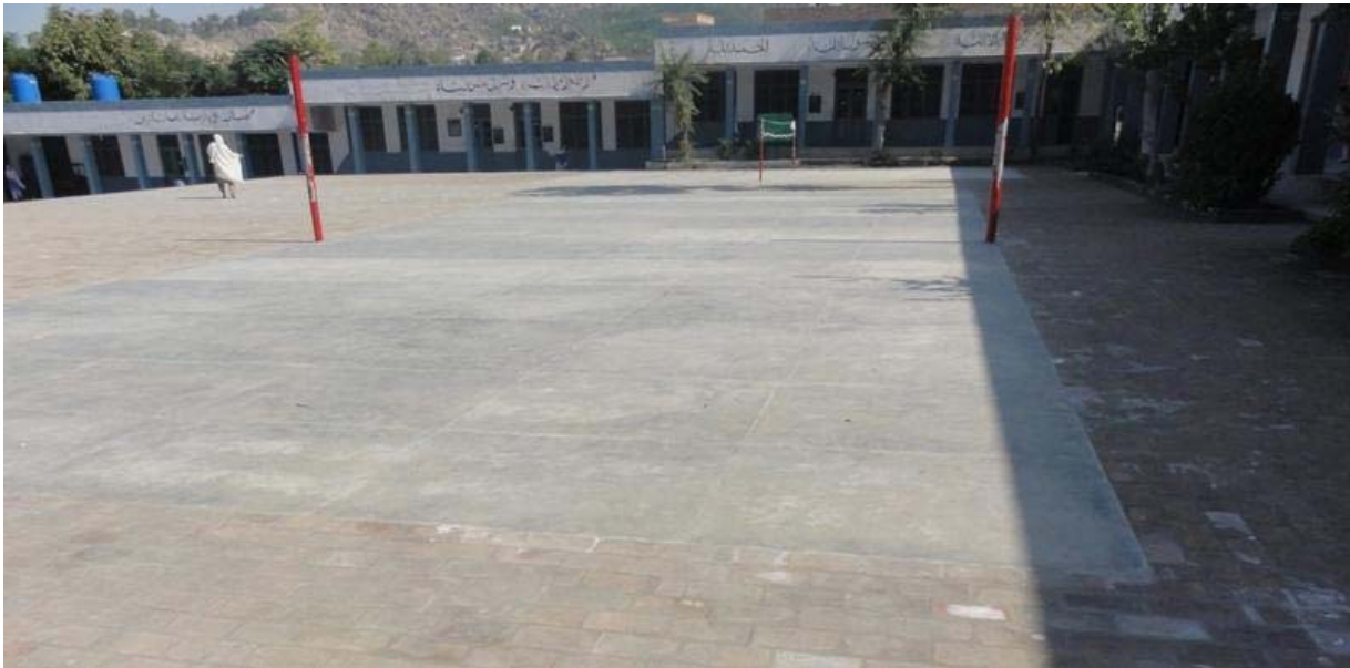
The Government Girls' High School, damaged during military operations, has been rehabilitated and is now open. (Photo by OIG, October 2011)
