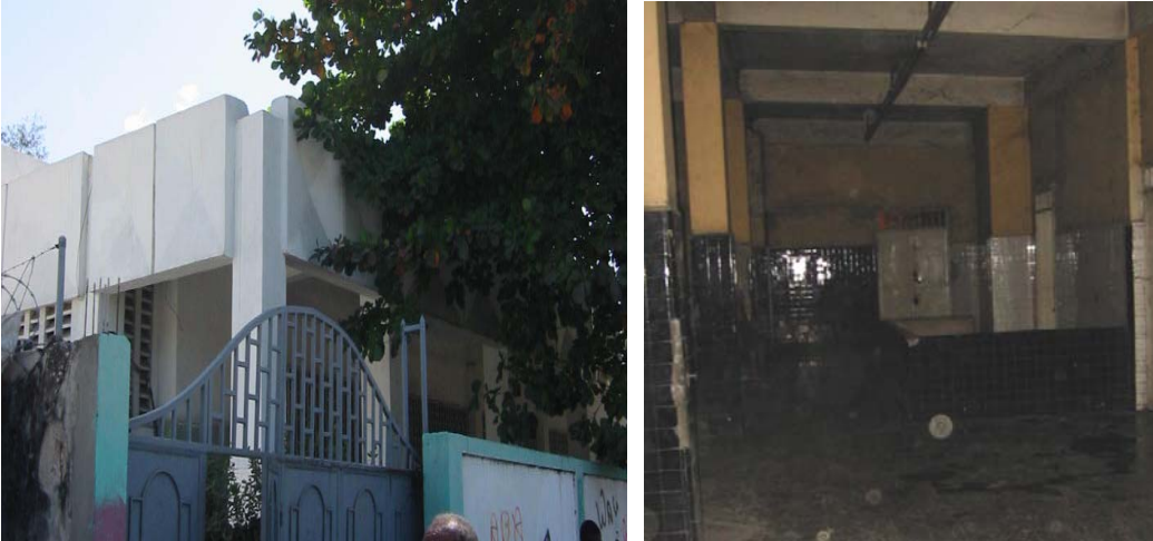
Photos taken by an OIG auditor on January 25, 2008 of the inside and outside of the site tentatively selected to be the parliamentary research center
