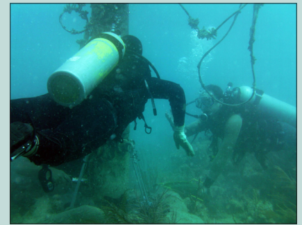
LTJG Rachel Kotkowski and LCDR Hector Casanova of AOML work to replace the spectra lines at the CREWS station in La Parguera, Puerto Rico.
