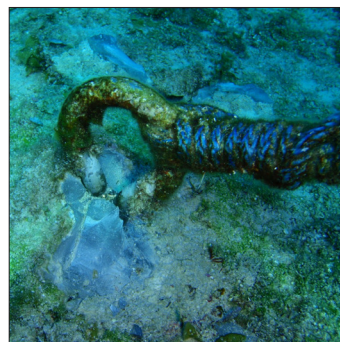
The concrete bed beneath one of the Little Cayman Island ICON station's peripheral anchoring pins appears to have sustained damage through cracking, attributed to the recent earthquake and aftershocks in the Caribbean.
