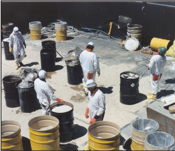
Removal of contaminated residue from the 183-H Solar Basin
