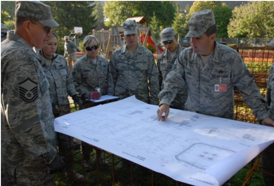
Master Sgt. Homer King, right, reviews a drawing with his team concerning rebar specifications on a concrete slab they poured.
