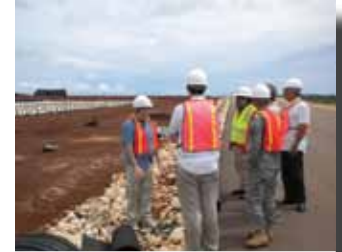
DoD IG team inspecting the new solid waste facility in Guam.
