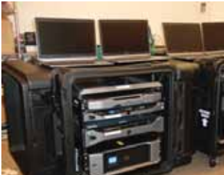
DCIS works with DMEN, a secure digital media-processing network.
