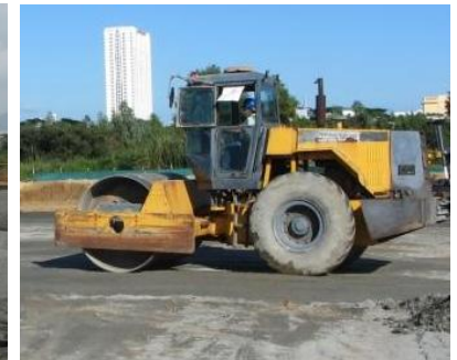
Compacting fill material (Photo: CDM Smith)
