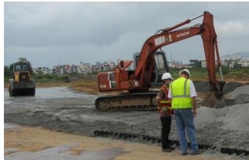
Importing clean, structural fill material (Photo: CDM Smith)
