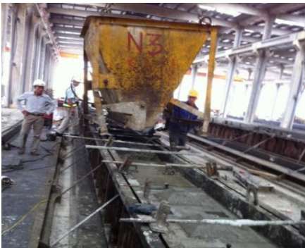
Pouring CMU blocks into molds (Photo: CDM Smith)
