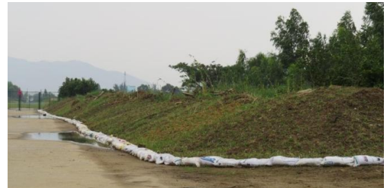
Stockpile of approximately 250 m 3 of clean topsoil material being composted (Photo: CDM Smith)
