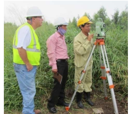
Surveying excavation limits (Photo: CDM Smith)
