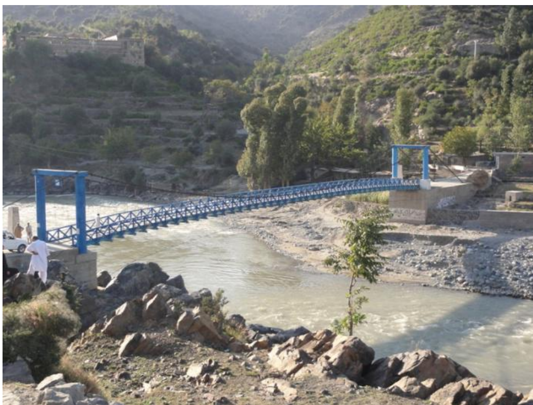
A bridge funded by the Pakistan Transition Initiative Program allows for quick and safe river crossing. (Photo by OIG, October 2011)
