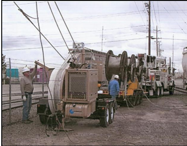
Photograph 2-9 Example of a Pulling Station
