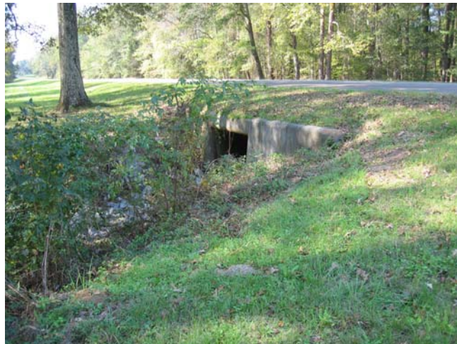
Figure 14. Site 2 culvert, near mile post 69.
