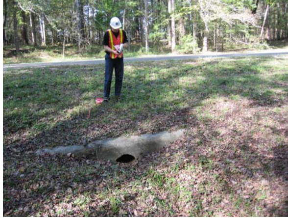
Figure 15. Site 3 pipe, near mile post 70.
