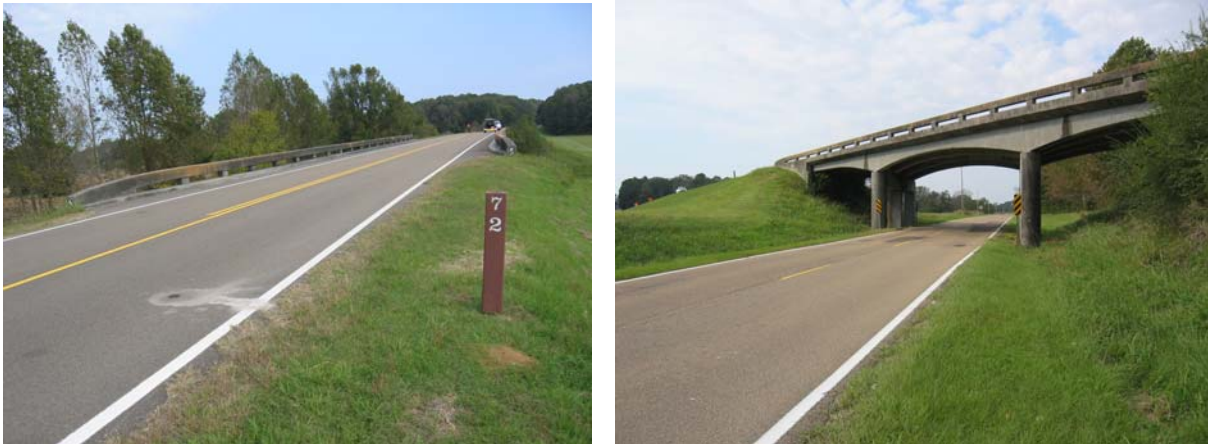
Figure 17. Site 5 bridge at mile post 72.
