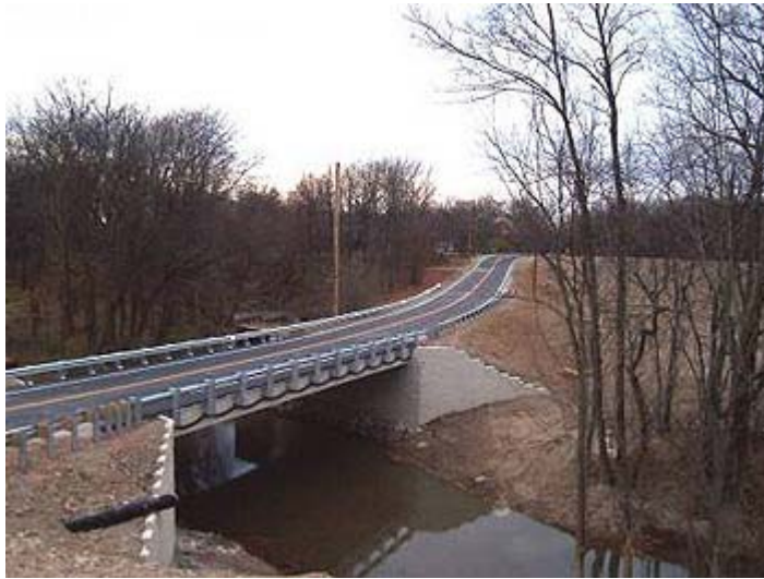
The completed Bowman Road bridge, located in Defiance County, Ohio. Although it looks very conventional, this bridge's abutments were constructed with GRS systems. There are five others in the County, constructed in much the same way.
