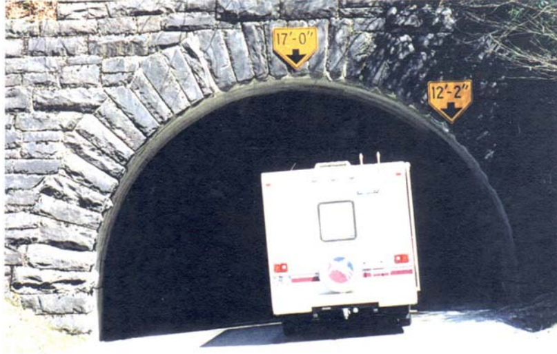
Figure 1. Condition prior to improvements – this is intended to be a two-way highway.
