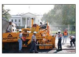
to have a unique rustic look. The mix design was originally conceived to resemble a dirt road and consisted of a polymer binder produced by Neville Chemical and brought in from Pittsburgh, PA. This special material was used in lieu of a traditional liquid asphalt binder. The course aggregate used for the mix was brought in from Maine and the pink quartzite sand from South Dakota.
