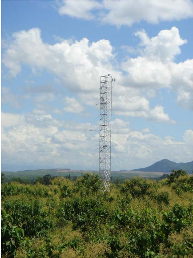
Figure 5: The tower in MMP.
