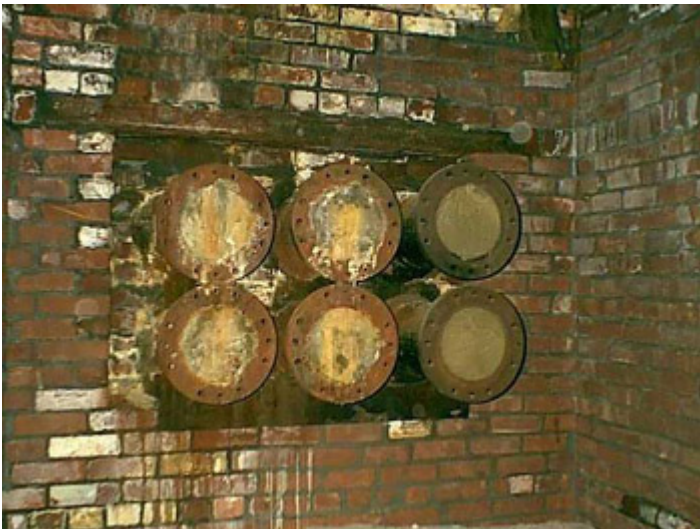
Figure 9. Flanges that are remnant tubes at Old Chelsea Street Postal Station.
