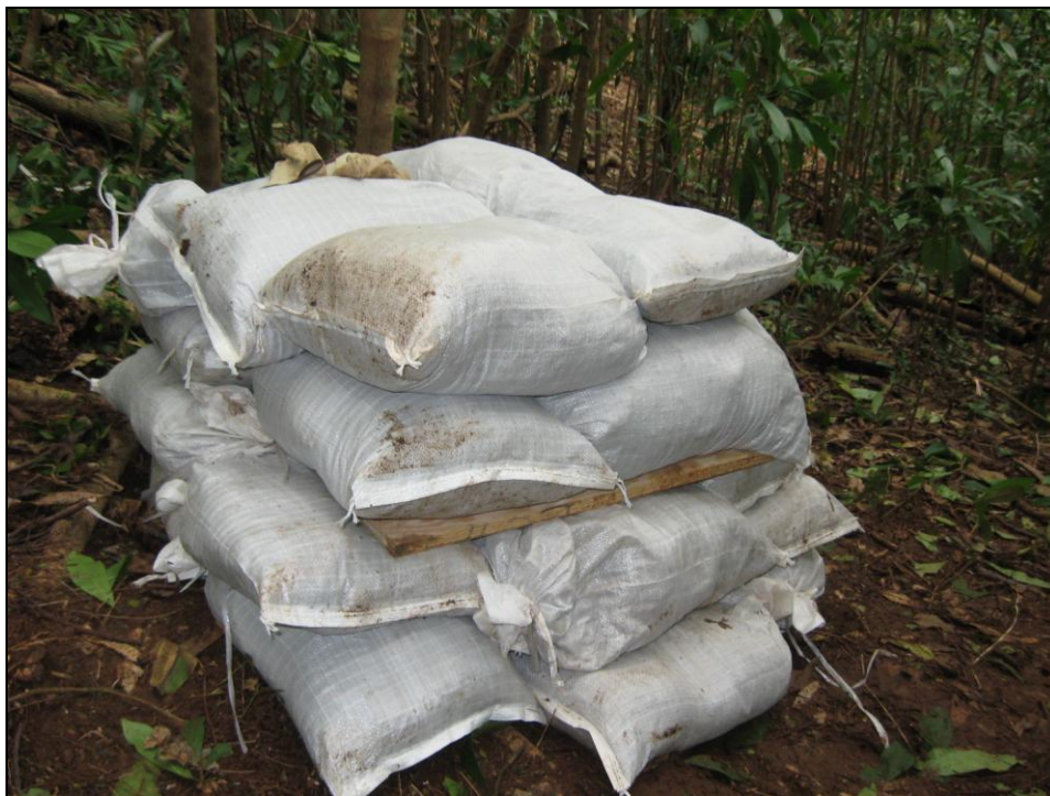
Photo 12 Protective Work with Sand Bags During Detonation
