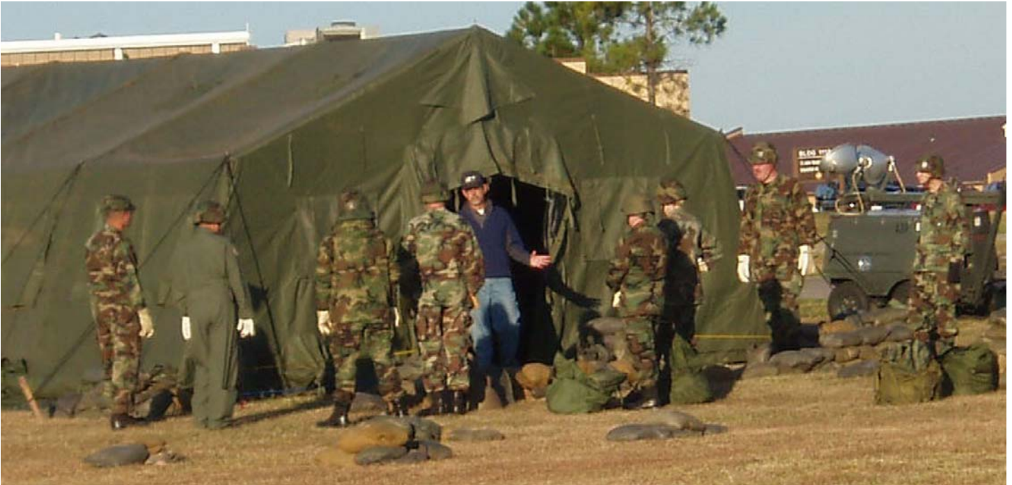
Mr. Jonny Conover, 72nd Air Base Wing Senior Exercise Evaluator, demonstrates how to use sandbags to harden a structure, thus protecting the occupants and equipment stored inside.
