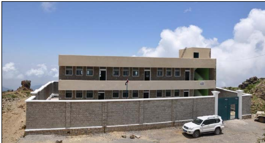
Before and after renovations of the Abdu Mohamed Al-Mekhlafe Scholl Zabid District, Hodeida Governorate (photos by USAID/Yemen).
