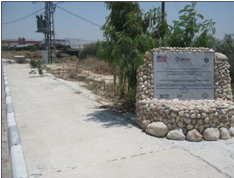
An Emergency Jobs Program plaque stands alongside the Beit Ur Al Tahta sidewalk project in the Ramallah Governorate (photo by OIG).
