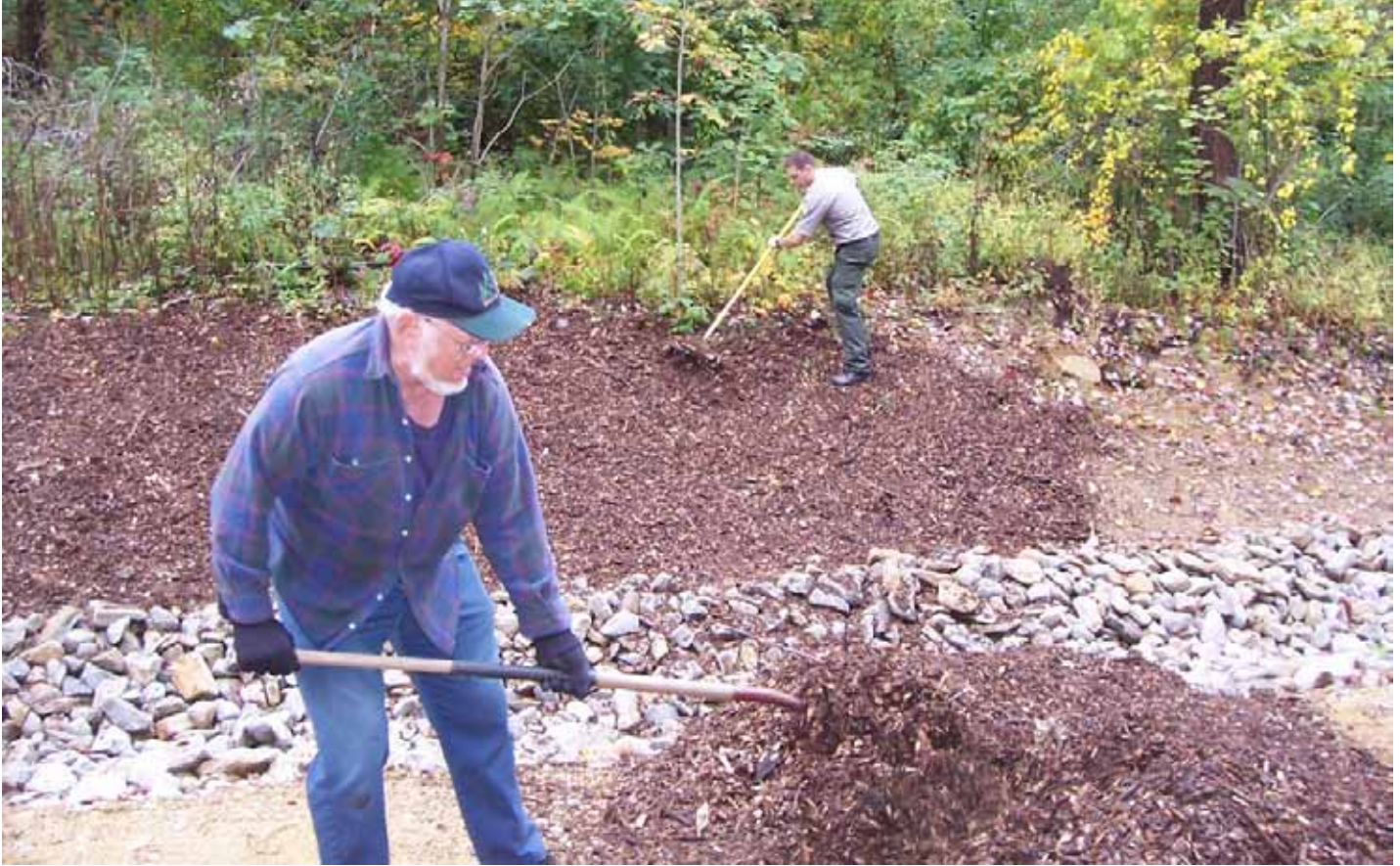
Volunteer Dick Caouette and Park Ranger Jesse Caney spread wood mulch for slope stabilization along the Heritage Trail in Southbridge.
