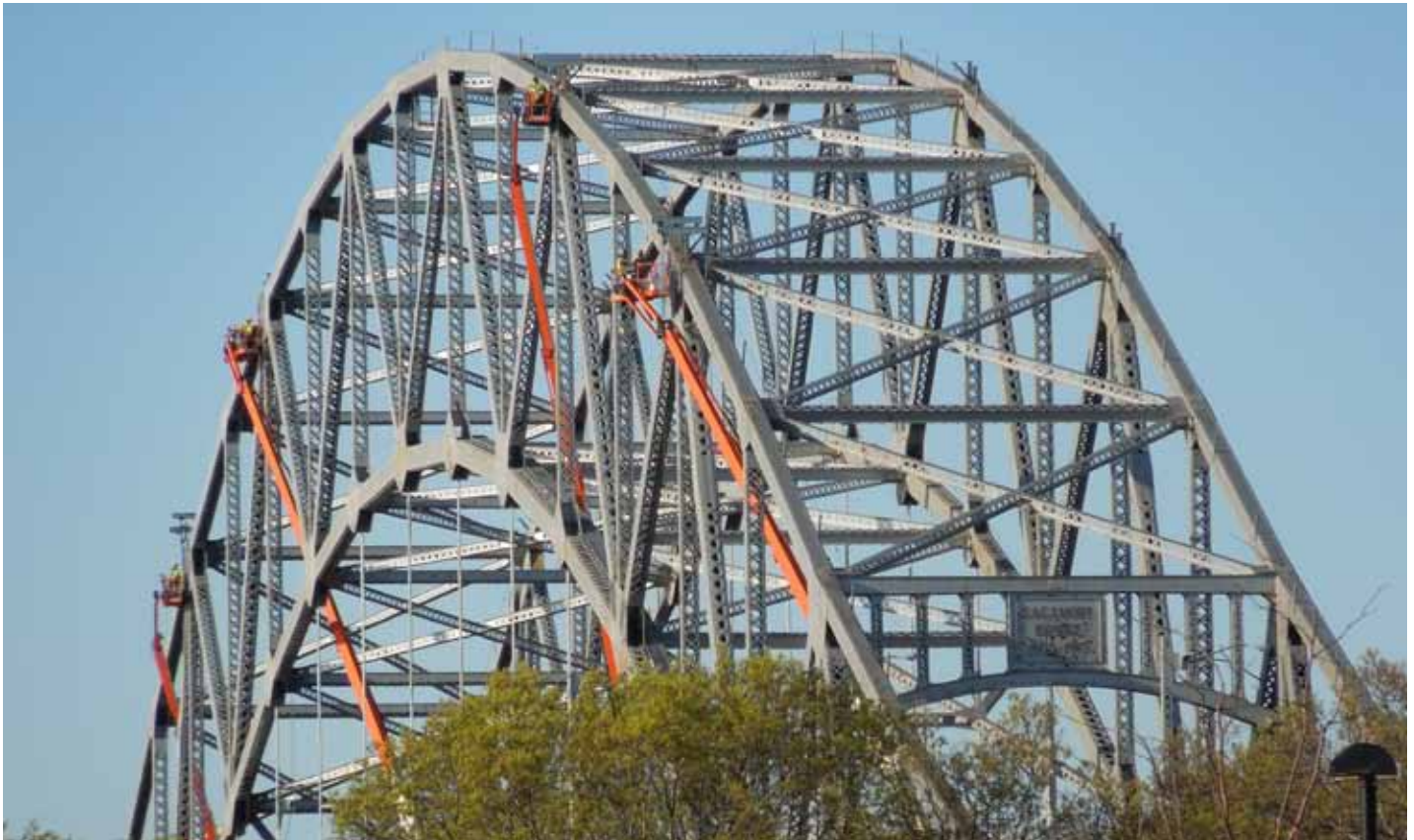
Repair work being performed on the Sagamore Bridge.
