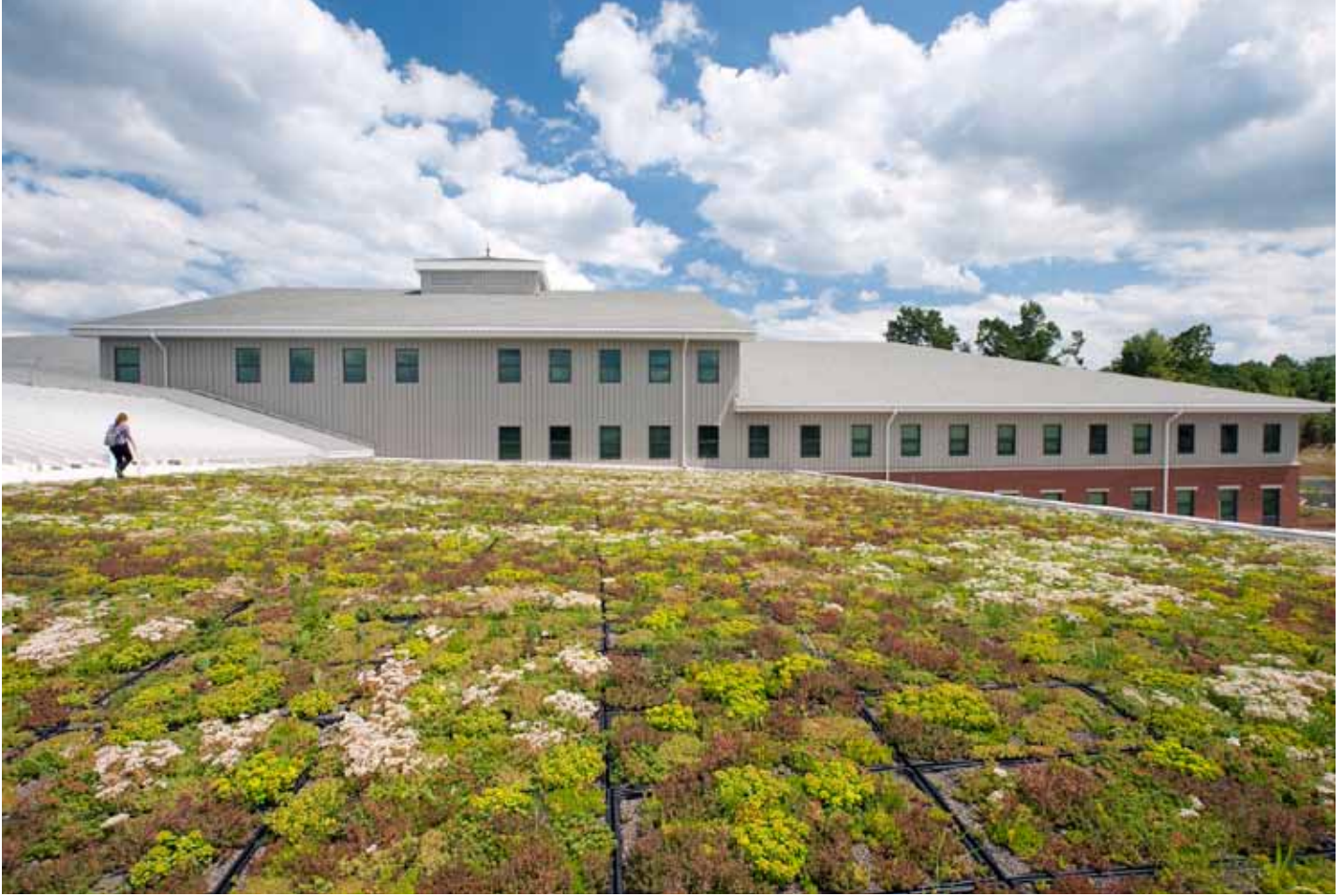
Vegetated roofing is only one of many environmentally friendly attributes to the Middletown AFRC.
