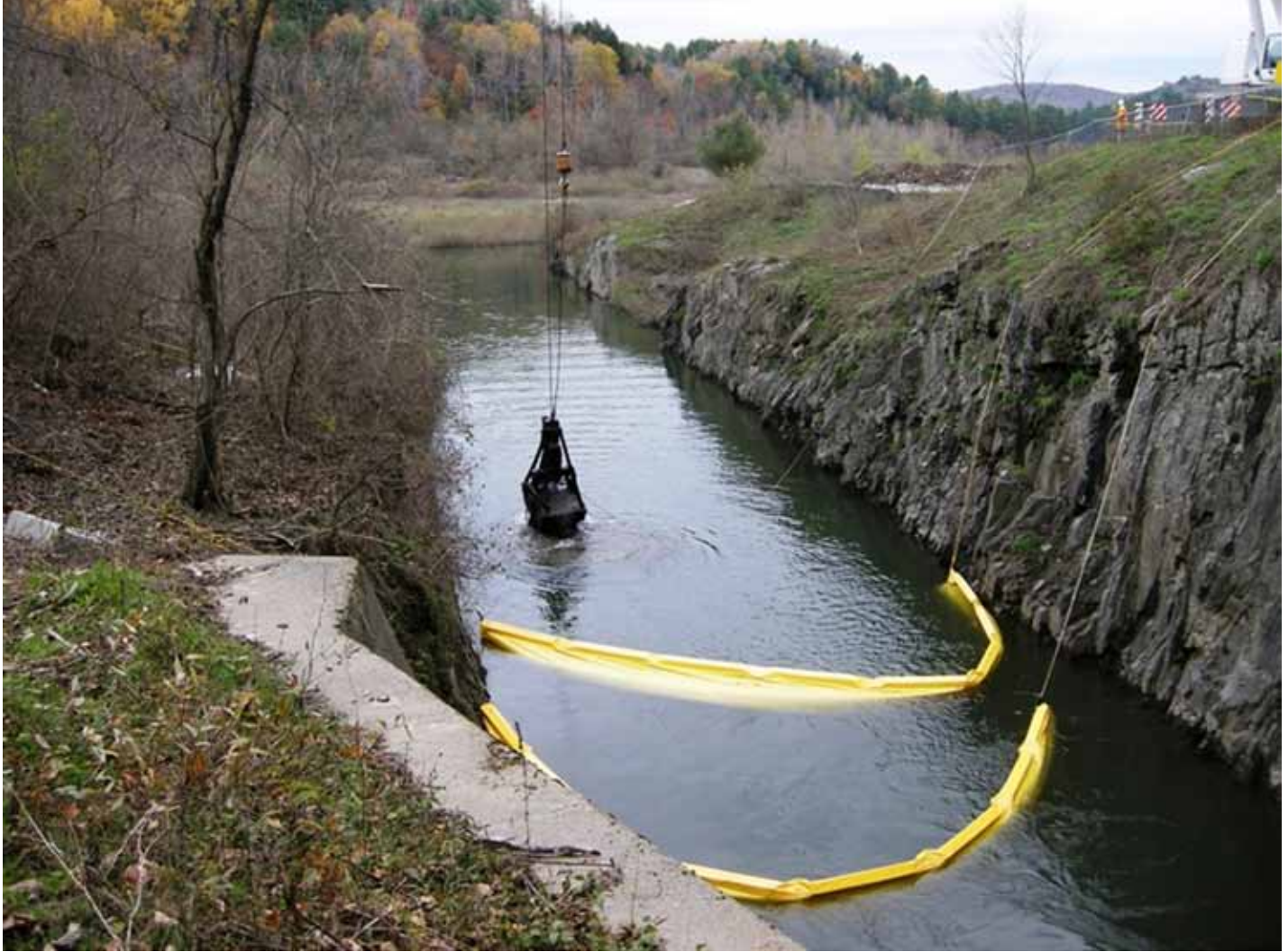
Contractor removes material from the intake channel at Union Village Dam.
