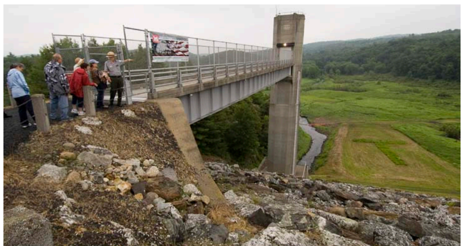
Thomaston Dam in Connecticut.
