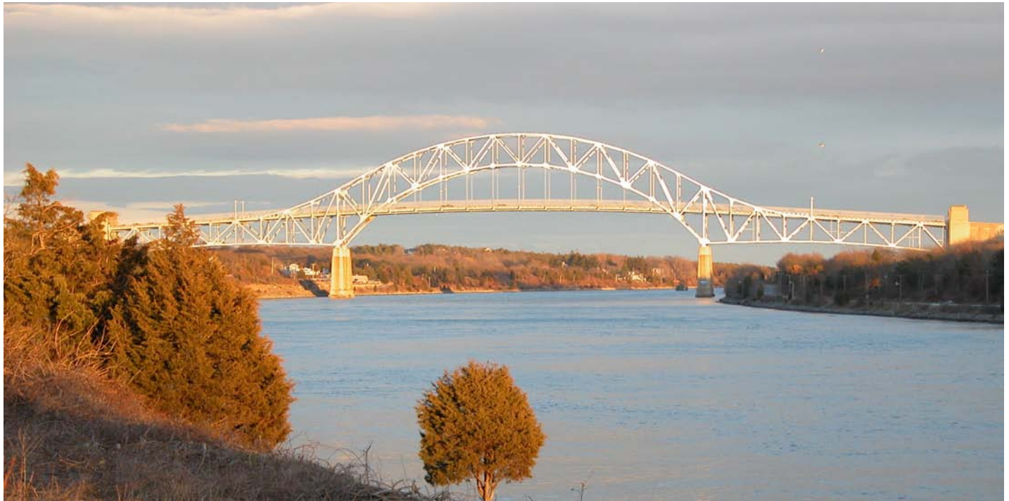
The Sagamore Bridge at the Cape Cod Canal in Bourne, Mass.
