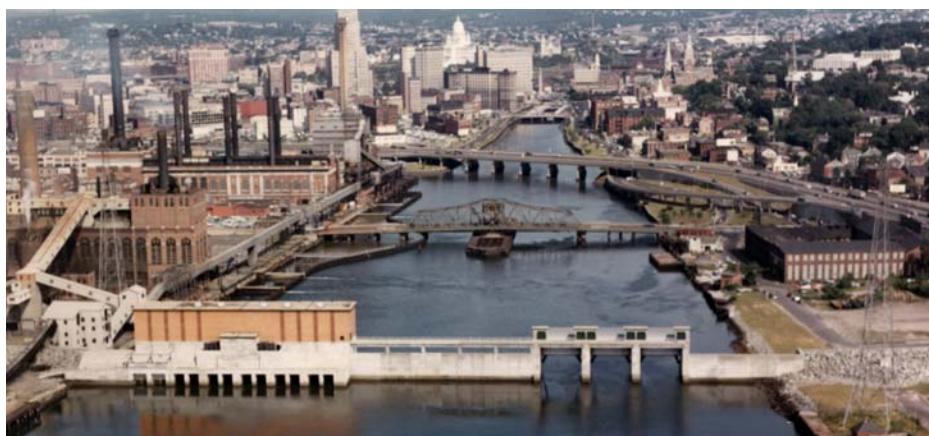
Fox Point Hurricane Barrier in Providence, R.I.
