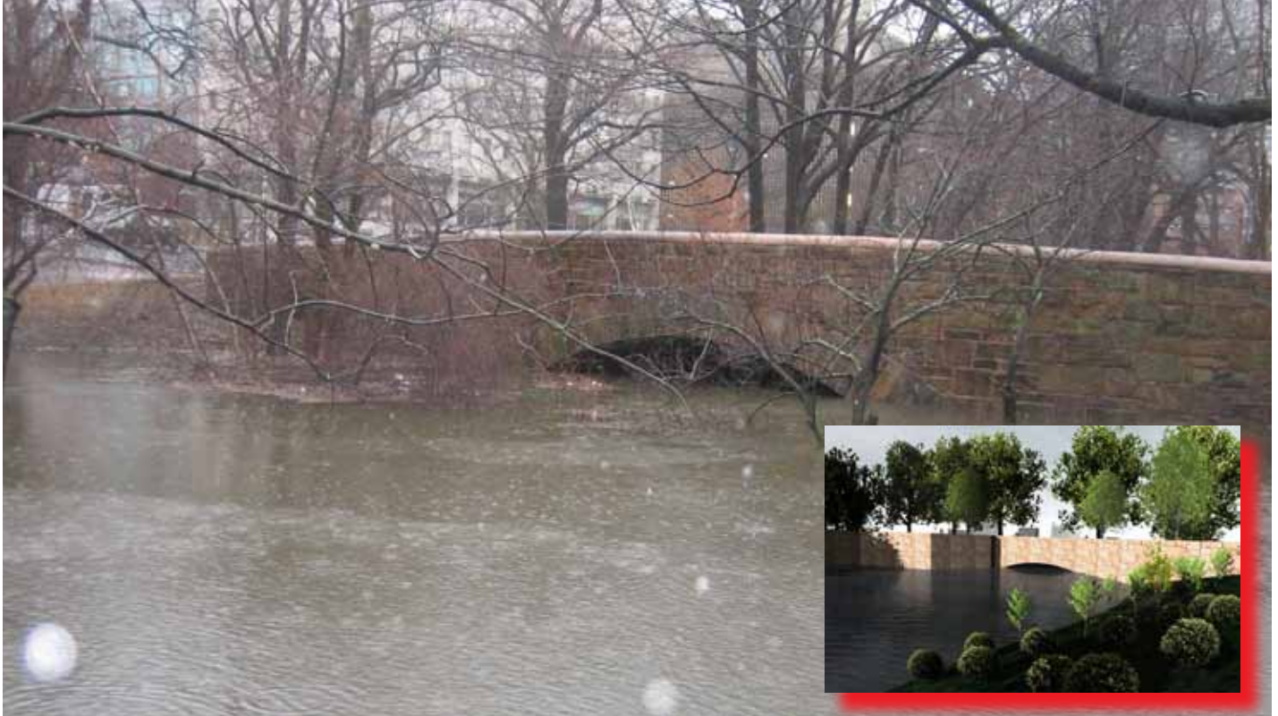
Flooding at the Netherlands Road Bridge. Inset: Artist rendition of a culvert set to be installed.
