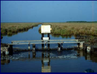
A weir controls water levels and salinity - Cameron Parish.
