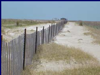
Sand fencing restores dunes on a barrier island - Terrebonne Parish.
