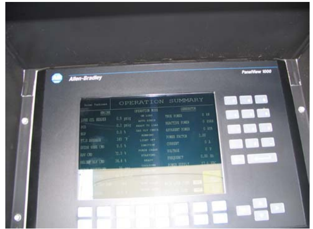
Figure 2.2 Allen-Bradley PLC – Main controller for the Mercury 50
