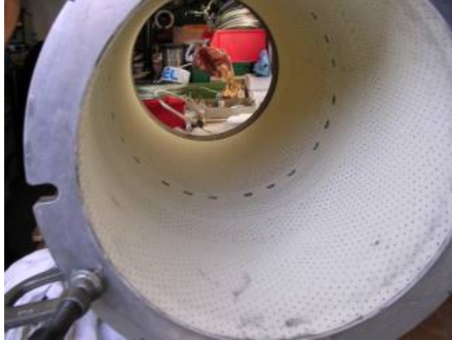
Figure 11. Interior View of the Axial Stage Transition
