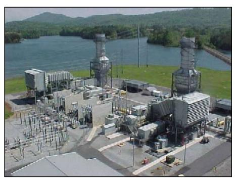
**Ashville plant.** Progress Energy peaking plant in Ashville, North Carolina is powered by two dual-fuel Fr 7FA units that served as in-service "test beds" for checking out development of the health management system.
