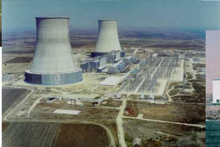
Natural Draft Circular Cooling Towers
