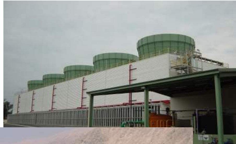
Mechanical Draft Wet Cell-Type Cooling Tower
