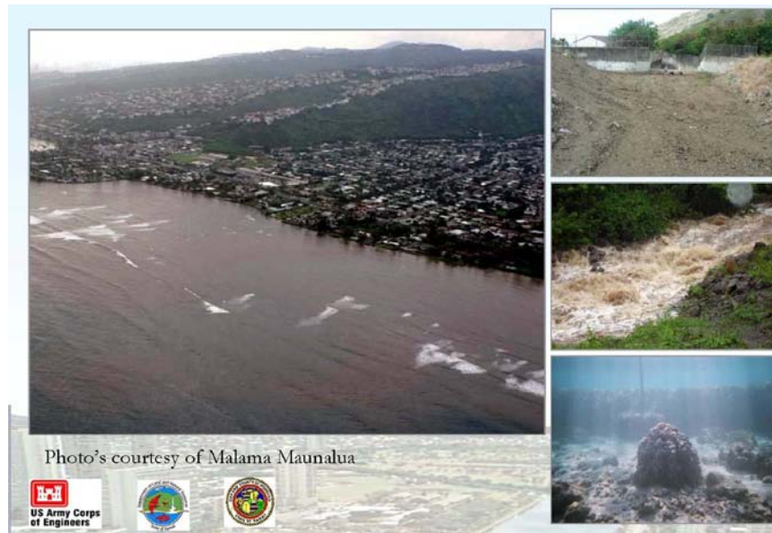
FIGURE F-6: MAUNALUA BAY EAST OF ALA WAI WATERSHED (TOP LEFT). EXAMPLES OF TRAPEZOIDAL CONCRETE CHANNELS DURING HIGH FLOW EVENTS (TOP RIGHT, MIDDLE RIGHT). CORAL REEF IMPAIRED BY SEDIMENT IN MAUNALUA BAY (BOTTOM RIGHT).
