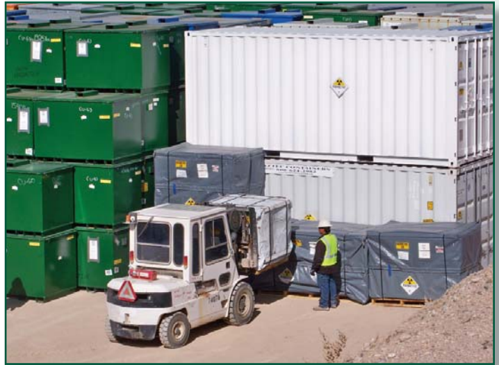
Waste packages are positioned for disposal in a disposal cell at the NNSS Area 5 Radioactive Waste Management Site
