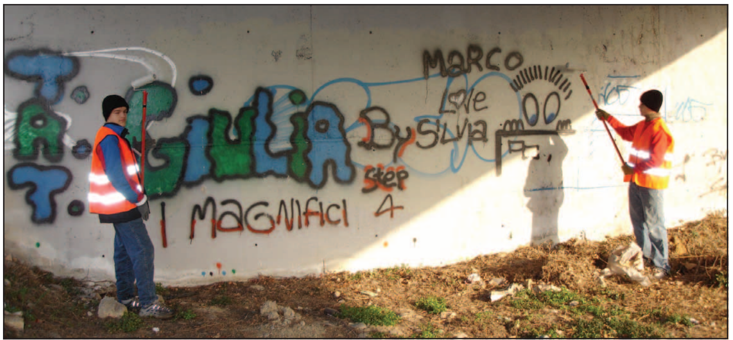
Boy Scouts from Troop 295 begin to paint over the graffiti on one of the bridge abutments for via Aldo Moro, located off the main entrance to Caserma Ederle. The Scouts, along with help from adult leaders, spent most of Dec. 16 clearing debris and painting over the graffiti that disfigured the columns as a service project. (Photo courtesy of David Eldredge)
