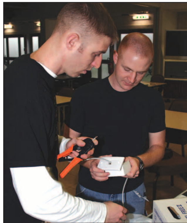
Sgt. Ryan Haraschack wires cable through a port with the assistance of Airman 1st Class Jason Woody. They are installing the new Xbox 360 system at the DCC.
