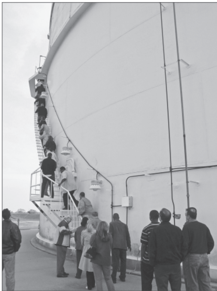
Participants in the Energy Indoctrination Course visit the marine bulk fuel terminal at Craney Island, Va.
