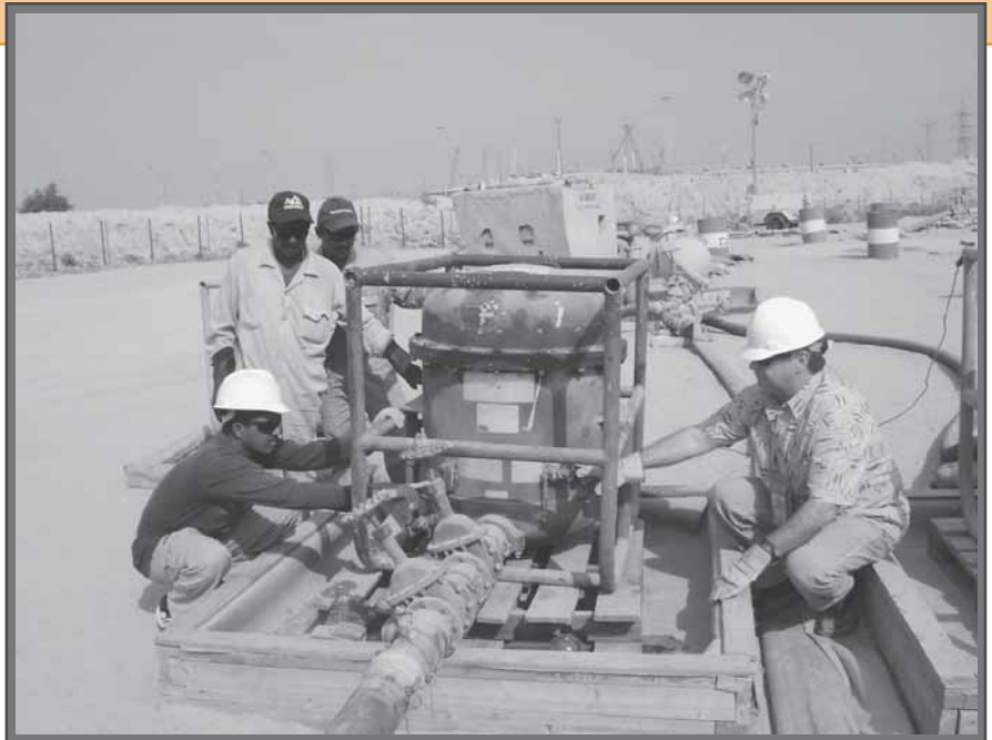
Quality Assurance Representative K.O. Williamson inspects a filter separator at a truck fill stand during a customer assistance visit in Kuwait.
