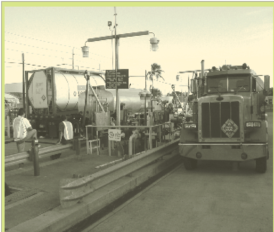
Fuel is transferred to the Iso-containers at the Fleet and Industrial Supply Center Pearl Harbor truck loading rack.
