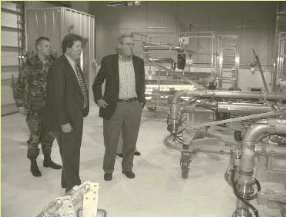
Norris, Larweth and Connelly view several of the new stainless steel pantographs purchased for Eielson AFB's new Type II hydrant system.
