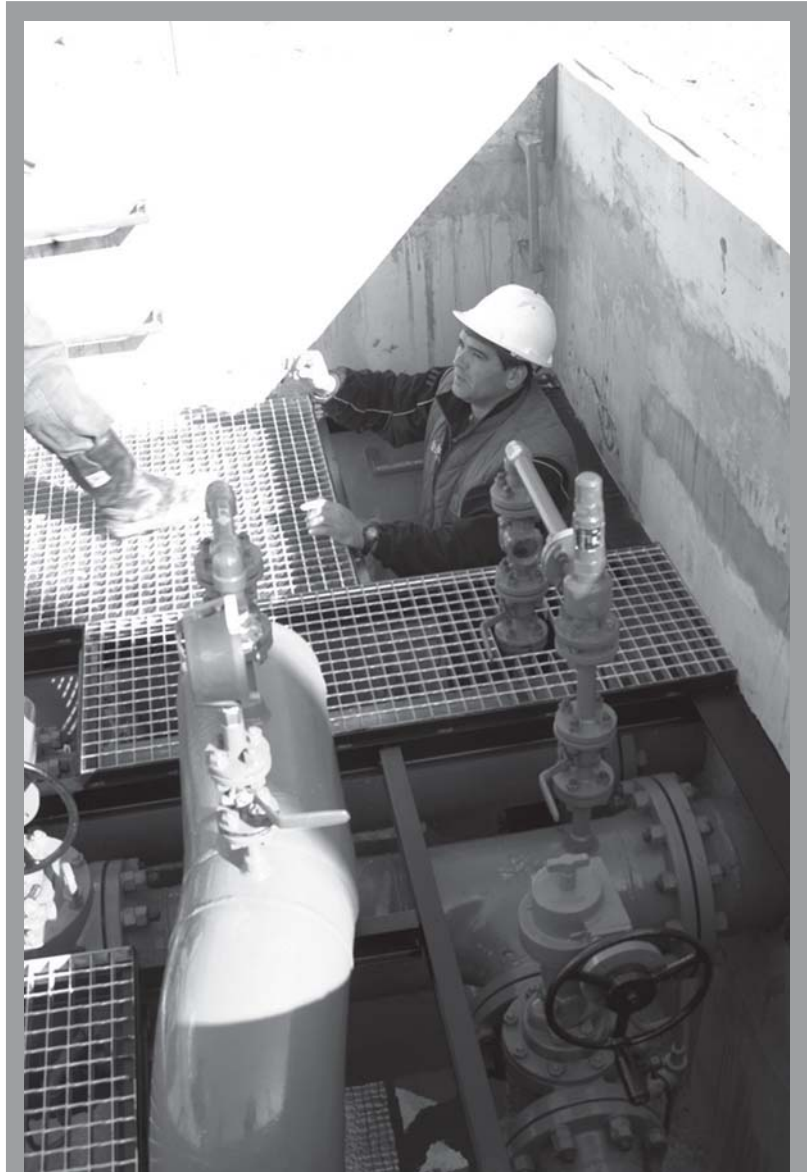
A worker toils in the valve pit area.
