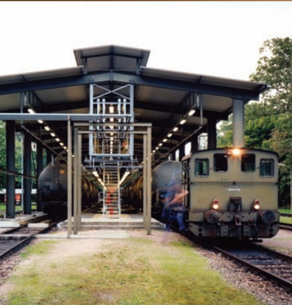
At a train loading station near the French-German border at Strasbourg, France, a railway tanker car is loaded with petroleum products. Photo courtesy of NATO.
