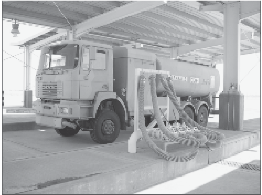
A fuel tanker positions to download fuel at the new Thumrait Air Base Tank Truck Offload Facility.
