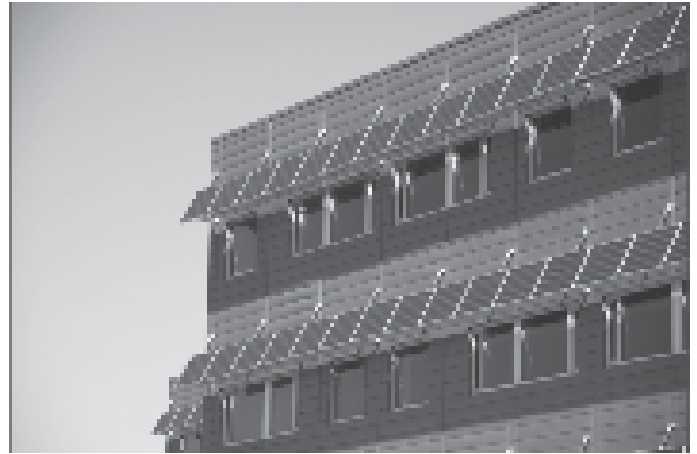
A building renovation capitalizes on environmental technology. The solar panels do double duty: they provide energy and shade. They collect energy for electricity and lower the ambient temperature within the building by shading the windows. (Courtesy photo)
