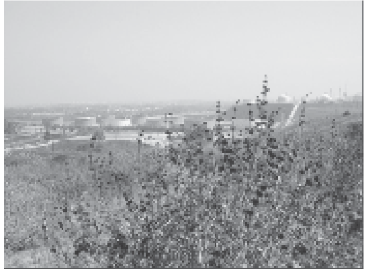
Defense Fuel Support Point San Pedro, Calif., is one of the sites that benefited from Defense Energy Support Center’s testing policy.
